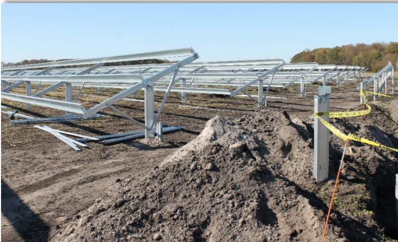
The new phase of the solar farm is under construction.
