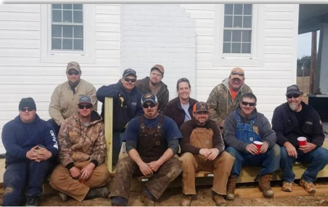
Employees of Mecklenburg Electric Cooperative take a break during construction of the wheelchair ramp they would finish later that day at their coworkers' home. (Photo: Priscilla Lawson Whirley)
