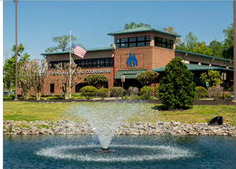
Choptank Electric Cooperative headquarters in Denton, Md.
